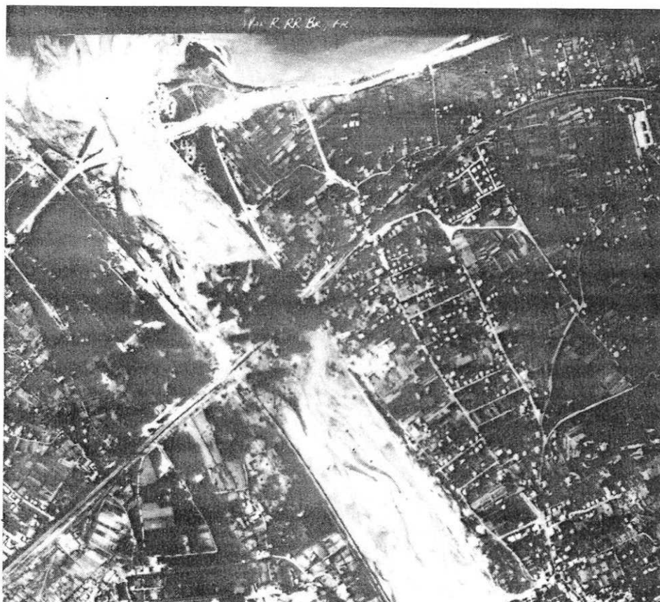
Var River R.R. Bridge, Nice, France June 7, 1944.
