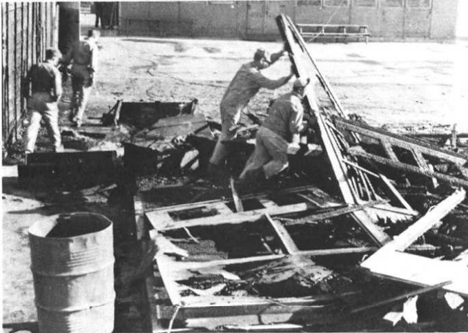
Army Engineers clearing rubble at Istres, France, June 1945.
