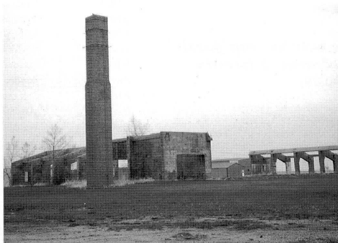
The burned out hangar at Harvard Army Airfield
