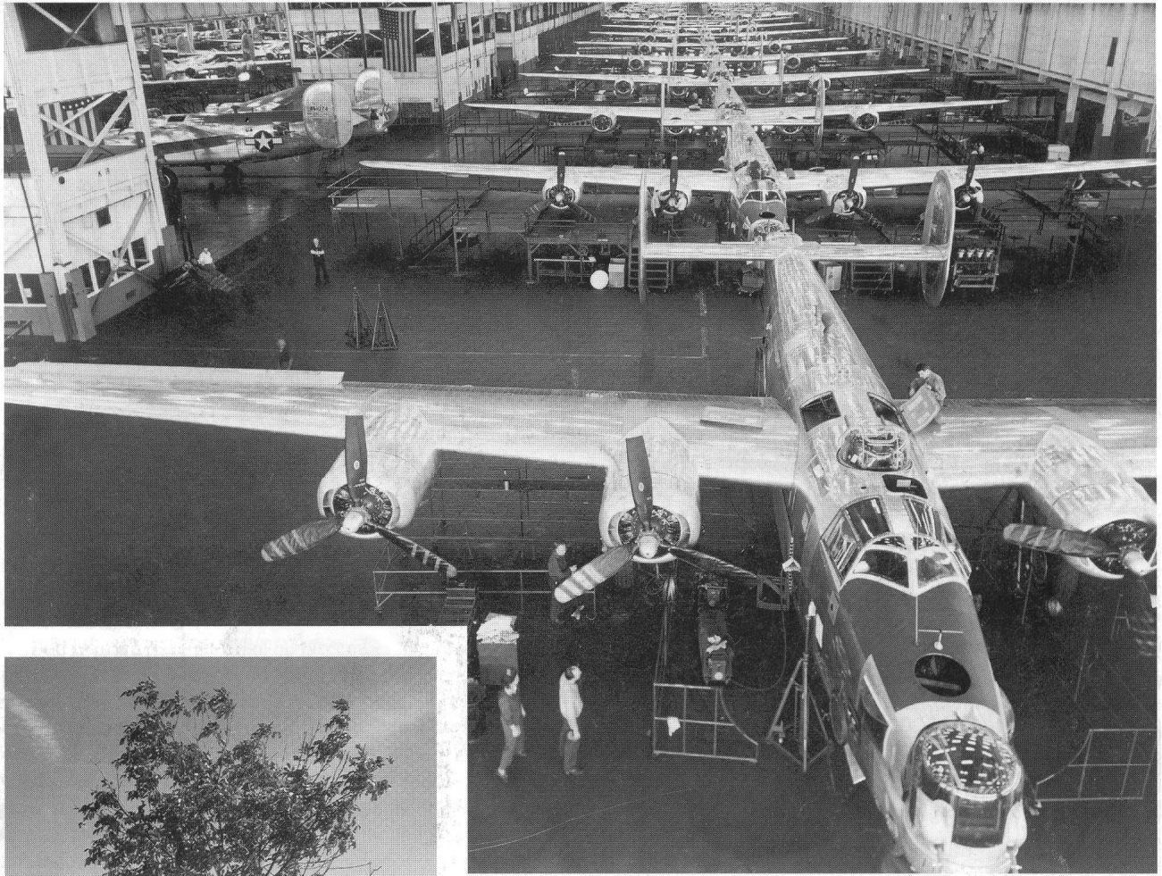
Photo above: Production of late model B-24s at the Ford Willow Run Bomber Plant. See Editorial page 38. Ford Archives/Henry Ford Museum, Dearborn, Michigan
