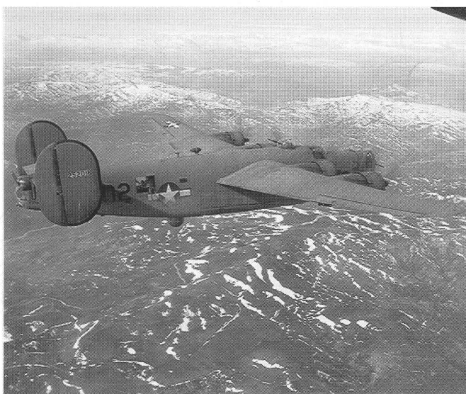
A typical "Mickey Ship" note the radome hung in the place of the ball turret.
