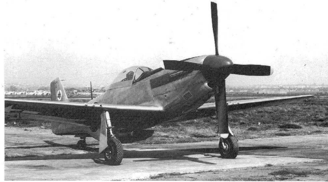
A P-51 showing the low air scope that led into the chamber producing the "Meredith Effect," See page 30.
